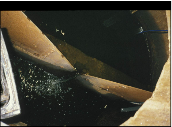
Modification of Outlet for Improved Performance
