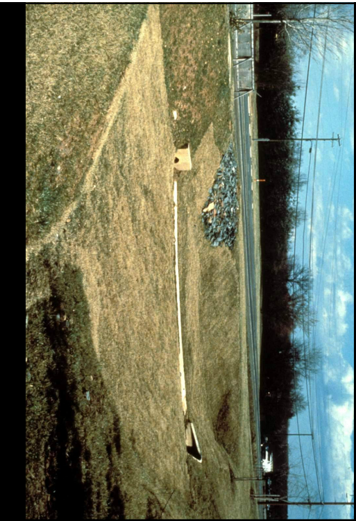
Typical Dry Detention Pond, with Pilot Channel
