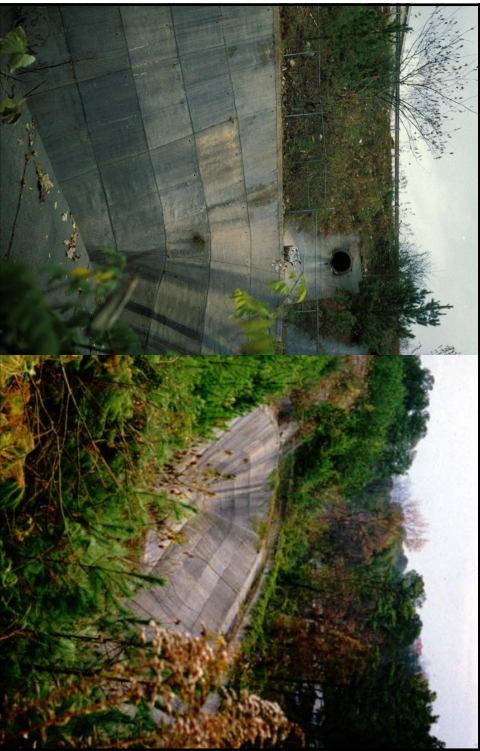
Unusual Dry Detention Pond Located on Hillside to Meet Peak Flow Rate Criterion
